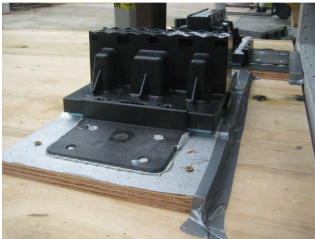
Prior to Exposure
